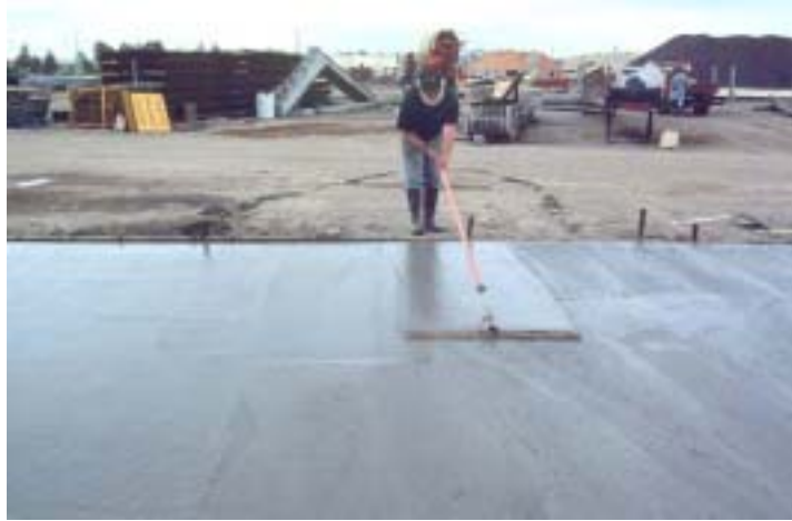
Fig 17. Finishing of cullet concrete
