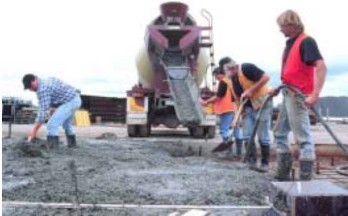
Fig 15. Placement of cullet concrete
