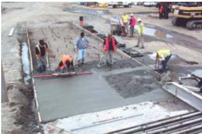
Fig 16. Finishing of section of glass cullet concrete
