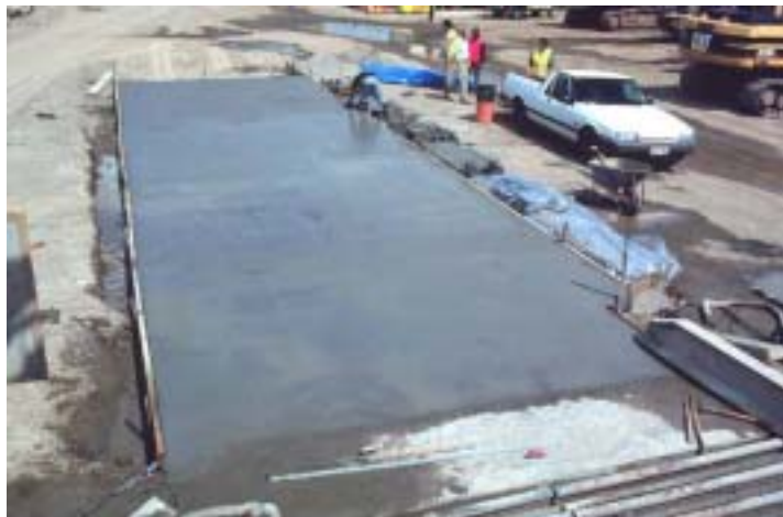
Fig 18. Finished cullet concrete for curing
